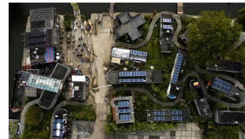
Fig 3.7. De Couvel, Amsterdam, aerial view of the project
